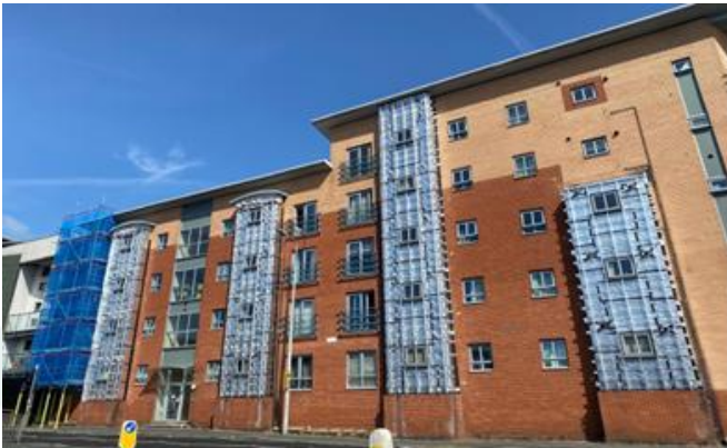
A photo showing Bracket and rails being installed
