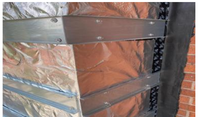
Progression on Elevation B
