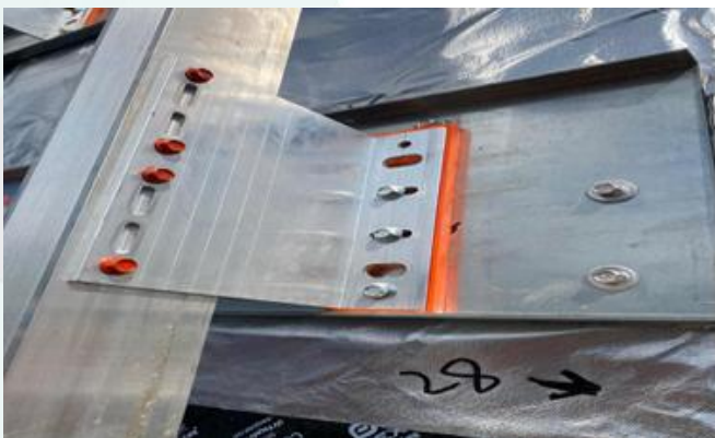
Progression on Elevation B
